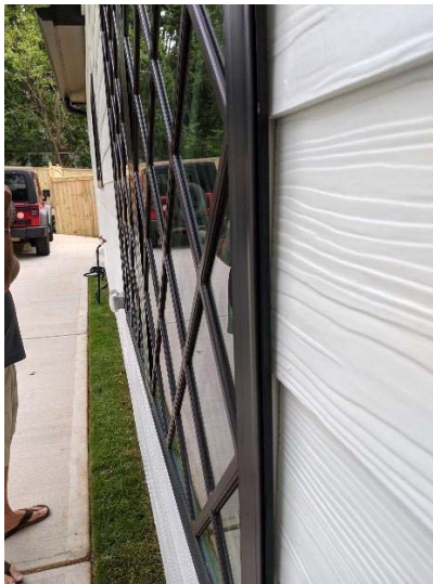
Multiple window showing trim, recession, and windowsills above. Trimmed out window per code below.
