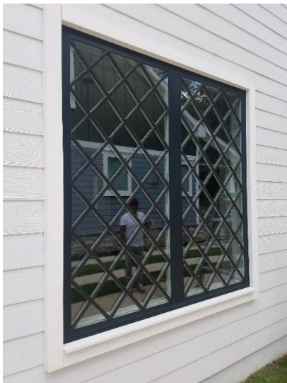
Multiple window showing trim, recession, and windowsills above. Trimmed out window per code below.
