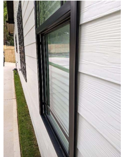
Multiple window showing trim, recession, and windowsills above. Trimmed out window per code below.
